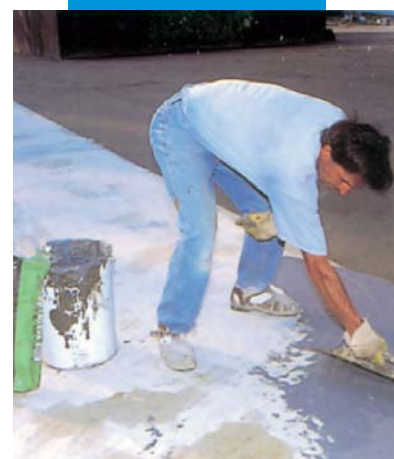
Hydroizolace bazénu Mapelasticem
